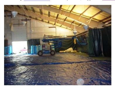
In May of 2006, we undertook the first of two major summer renovations, the replacement of our ceiling insulation system on courts 5 & 6. We first had to tear down all the existing insulation, and performed that task in house. We then hired Commercial Retrofit out of Michigan come in and install the new insulation.
